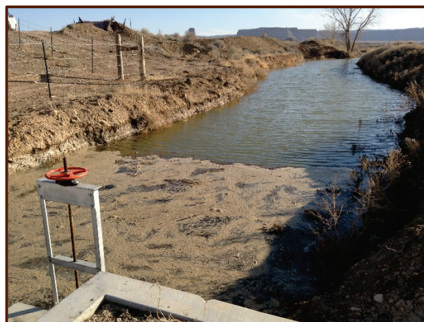
Mancos Creek Farm Ditch Source: Ute Mountain Ute Tribe
