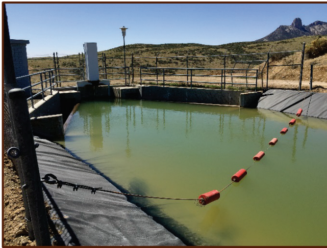
Canal siphon at the foot of Sleeping Ute Mountain Source: Ute Mountain Ute Tribe
